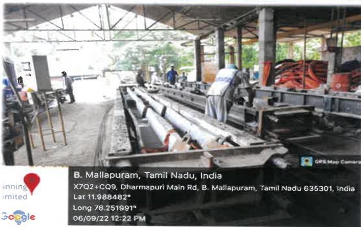
Railway sleeper Manufacturing Plant – Bommudi, Dharmapuri.
